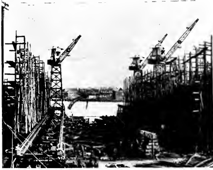
View of building berth showing tracks for electric tower cranes.
